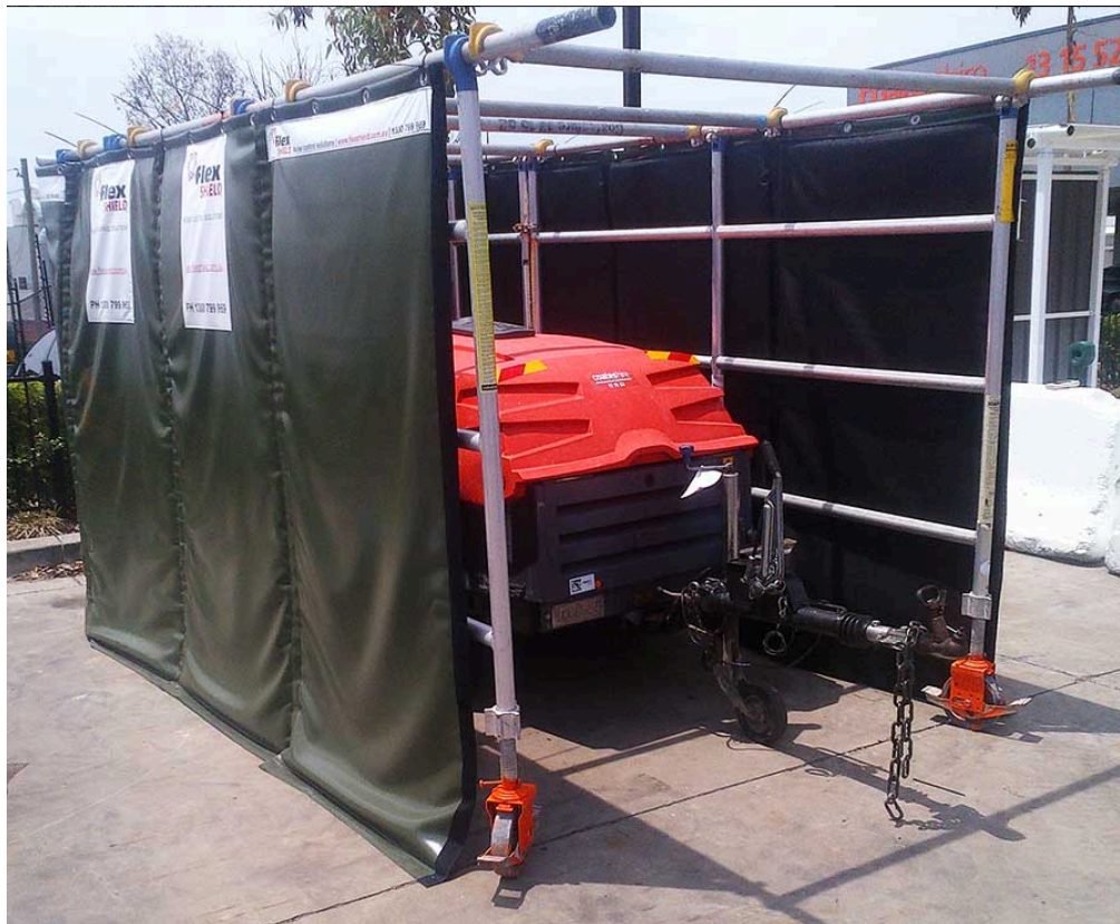
Figure 3 Example of a demountable noise barrier (Photo from Flexshield.com.au)
