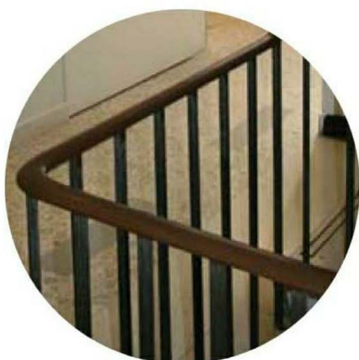
HR3 - HANDRAIL TYPE 3 BRONZE HANDRAIL (TO MATCH EXISTING) LOCATION: RELOCATED FIRE STAIR DESIGN INTENT: ECHO OF THE ORIGINAL STAIR
