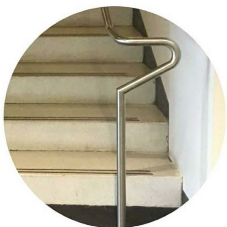
HR2 - HANDRAIL TYPE 2 STAINLESS STEEL HANDRAIL LOCATION: NEW INTERNAL HANDRAILS DESIGN INTENT: TO MATCH EXISTING
