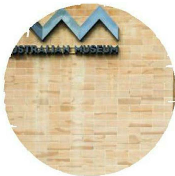
EXTERIOR SANDSTONE CLADDING LOCATION: FACING TO PARKES FARMER WING DESIGN INTENT: TO MATCH THE EXISTING HERITAGE FACADE
