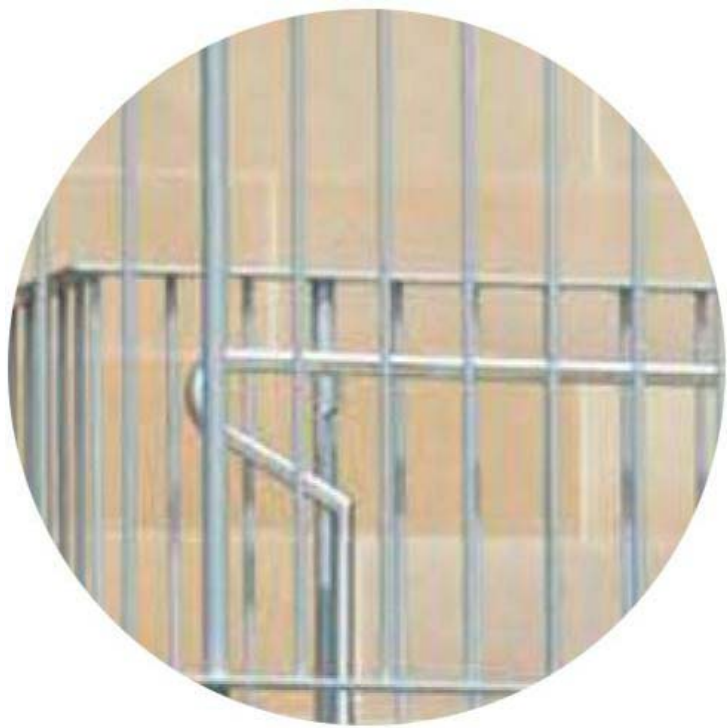
HR1 - HANDRAIL TYPE 1 PALLISADE STYLE BALUSTRADE AND HANDRAIL (TO MATCH EXISTING) LOCATION: ALL EXTERNAL HANDRAILS DESIGN INTENT: LIGHT AND FLIGREE, IN CONTRAST TO THE MASS OF STONE
