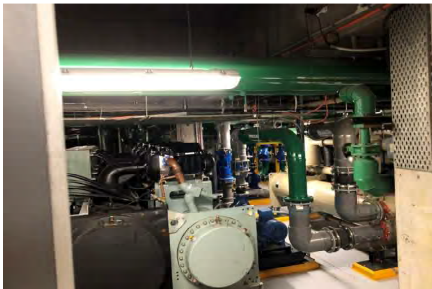
Photo 5 - Gas fired Air conditioning in Plant room 1
