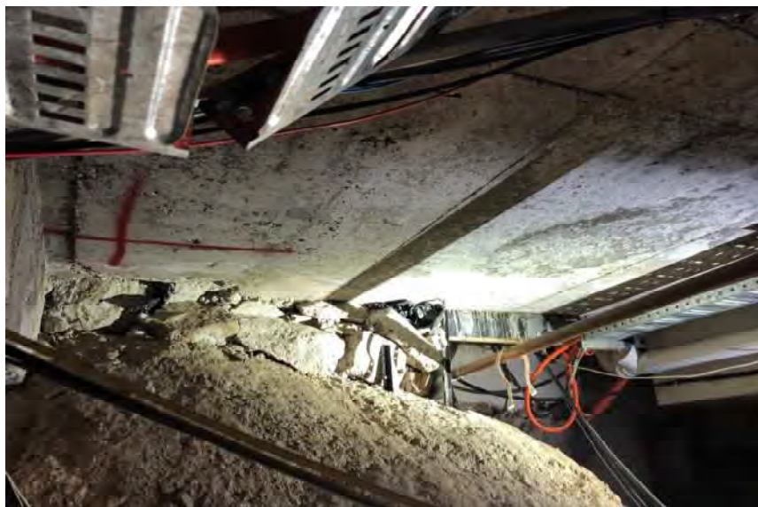
Photo 11 - Slab under Lewis Wing showing fill under slab
