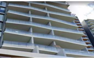
13 Courtyard Fritted Glass Balustrade
