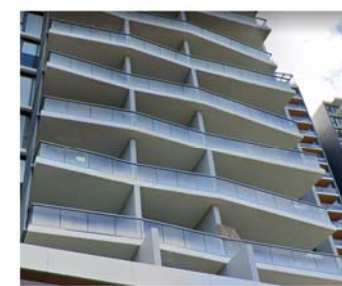
13 Courtyard Fritted Glass Balustrade
