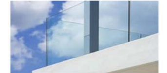
04 Clear Balustrade Glazing
