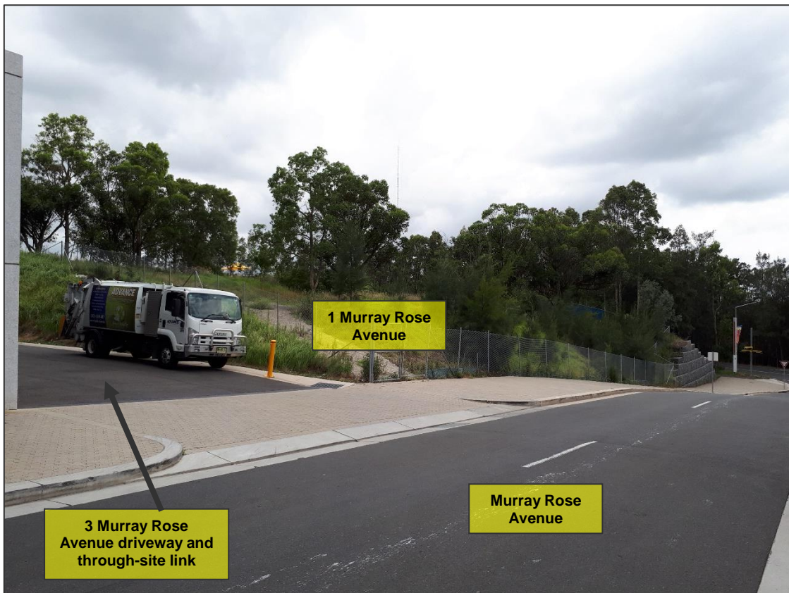
Figure 5 | 1 Murray Rose Avenue viewed from Murray Rose Avenue looking north-east (Base source: Department’s photograph)
