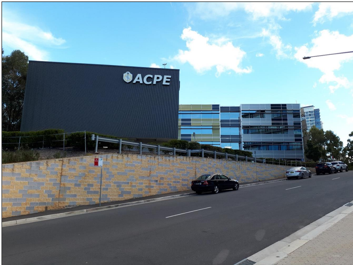
Figure 28 | Existing commercial building at 10 Parkview Drive (Source: Department's photograph)
