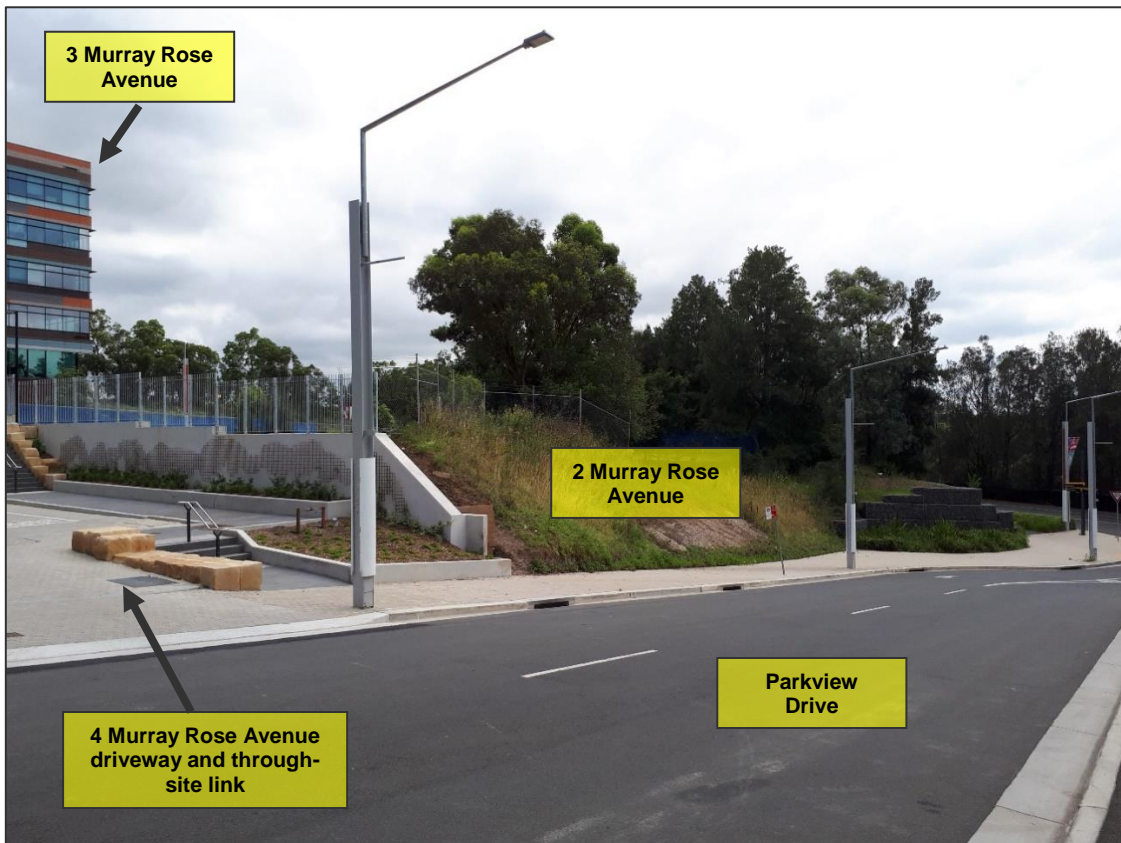
Figure 8 | 2 Murray Rose Avenue viewed from Parkview Drive looking north-east (Base source: Department's photograph)
