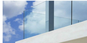
04 Clear Balustrade Glazing
