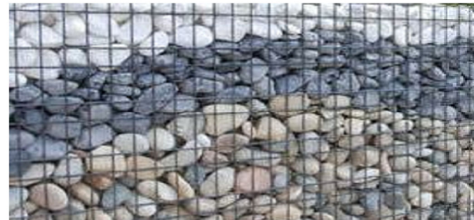
11 Gabion Feature Wall Finish or Similar
