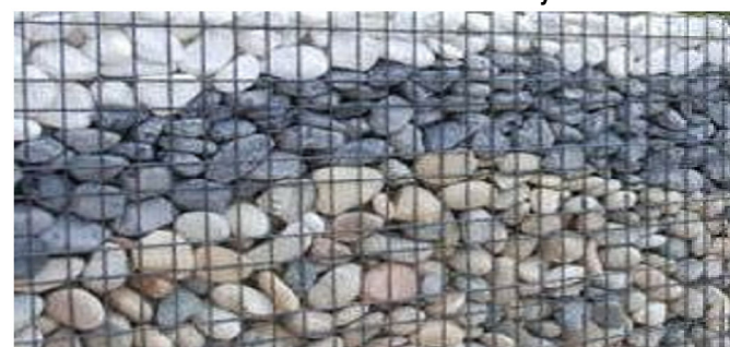
11 Gabion Feature Wall Finish or Similar
