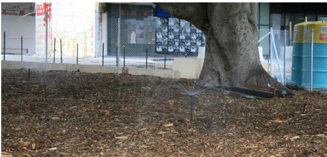
Figure 13 – Example of an automatic and battery operated irrigation spray system during construction (Image by Arterra 19/06/19).
