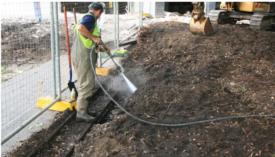
Figure 14 – Example of roots being non-destructively exposed using water jetting (Image by Arterra 06/06/13).
