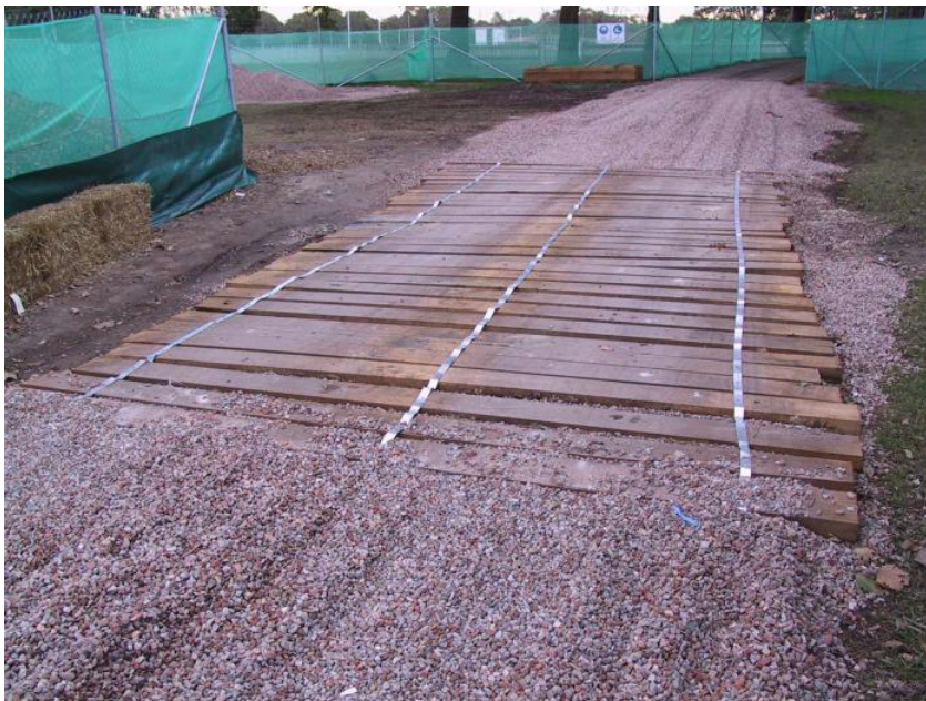
Figure 16 – Example of acceptable Tree Protection Area ground protection
