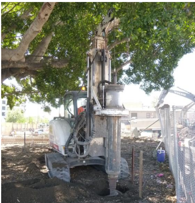
Figure 20 – Example of low height piling equipment being used under a Fig tree at Westfield Miranda (Image By Arterra 09/10/13)
