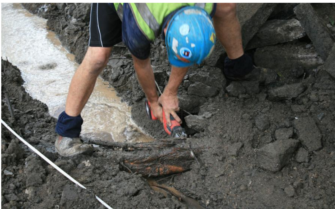
Figure 15 – Example of cleanly cutting exposed roots (Image by Arterra 06/06/13).
