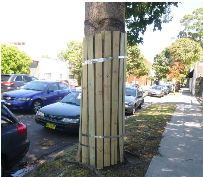
Figure 17 – Example of acceptable Trunk Protection batten installation
