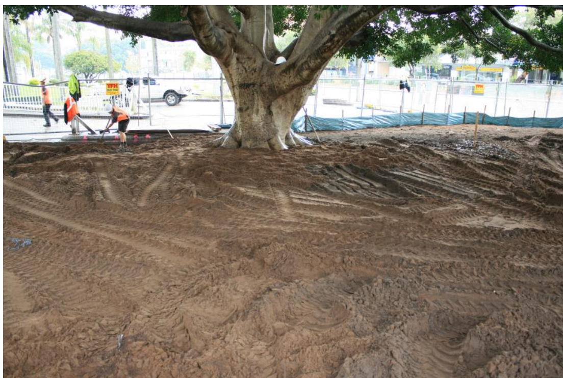
Figure 21 – Example of 100-200mm of new top soil spread under a Fig tree at Westfield Miranda (Image by Arterra 09/10/13)
