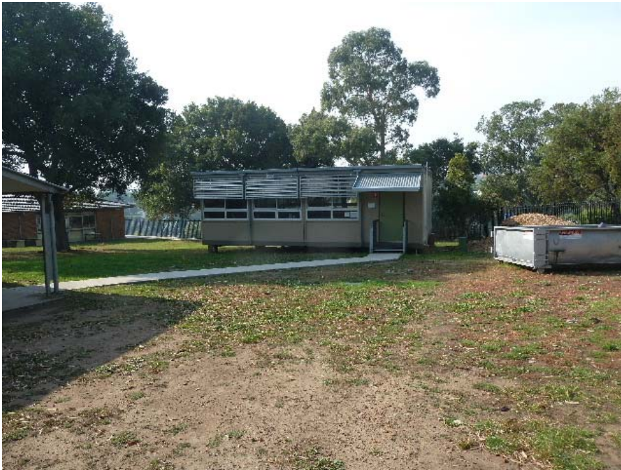
Figure 9: Exposures in project area
