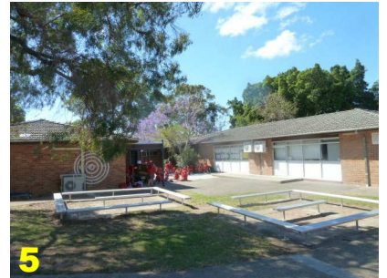
DISCONNECTED COURTYARD AREAS
