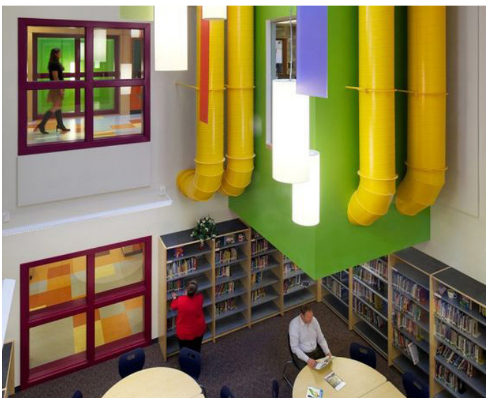
Colour Coded Services Pips
