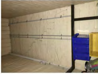
CRACKING TO WALLS IN BUILDING E (HERITAGE ITEM)
