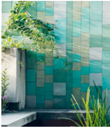
Tones of greens to metal cladding with expressed shadow gap joints
