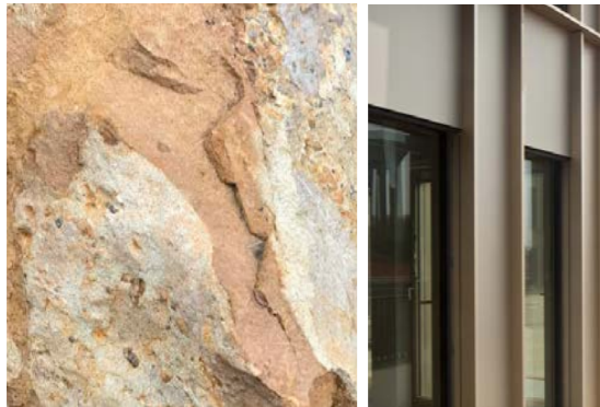
Standing Seam cladding articulated around windows
