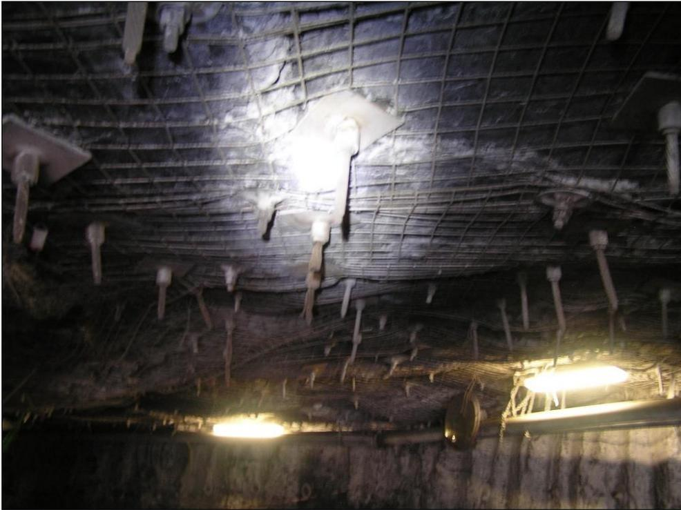
**Figure 17B – Underground Strata Conditions and Induced Damage due to Previous Surface Blasting (after ESC Study 2008)**
