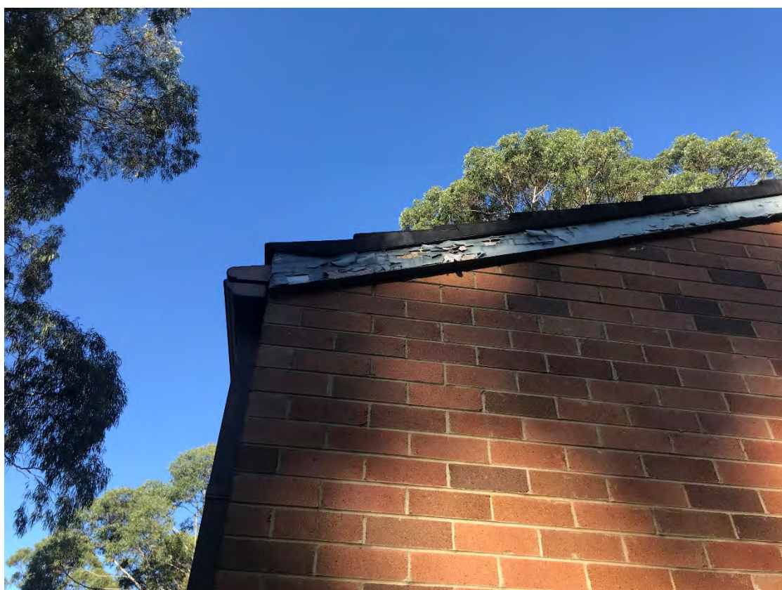
Photograph 4: Flaking paint on roof timber beams, which may potentially contain lead.
