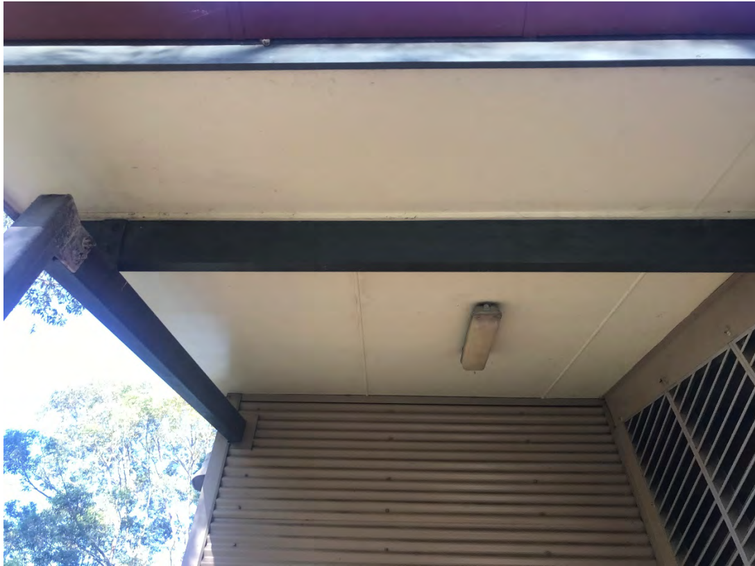
Photograph 1: Fibre cement sheeting (suspected to contain asbestos) identified within most building awnings.
