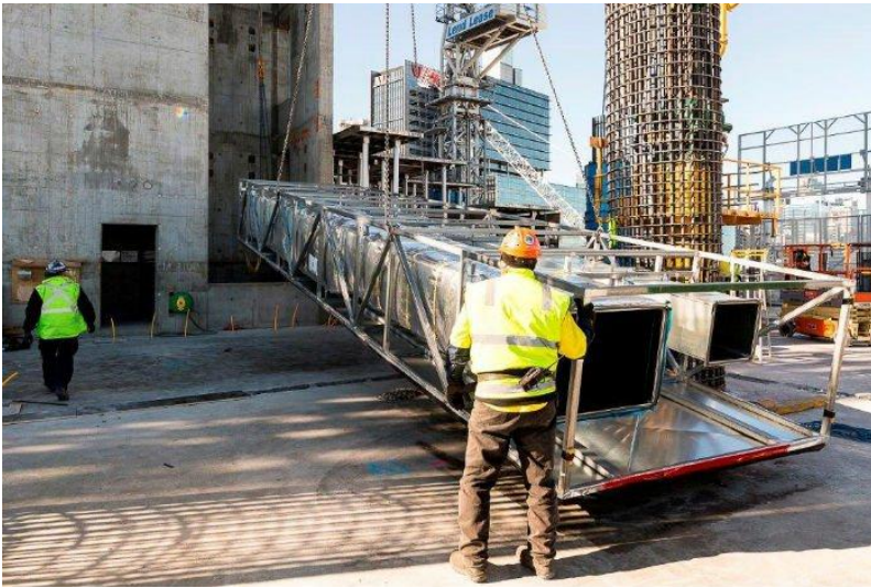
Figure 25 – Pre-fabricated Ductwork to Services Risers
