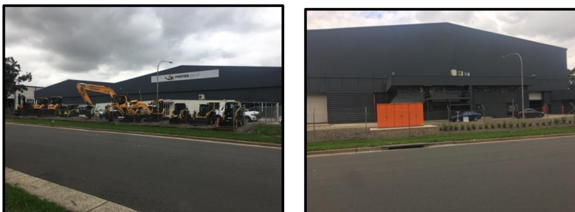
Figure 4: [left] Warehouse A [right] Warehouse B; as viewed from Loftus Road (Source: Concise Planning Pty Ltd, 2020)
