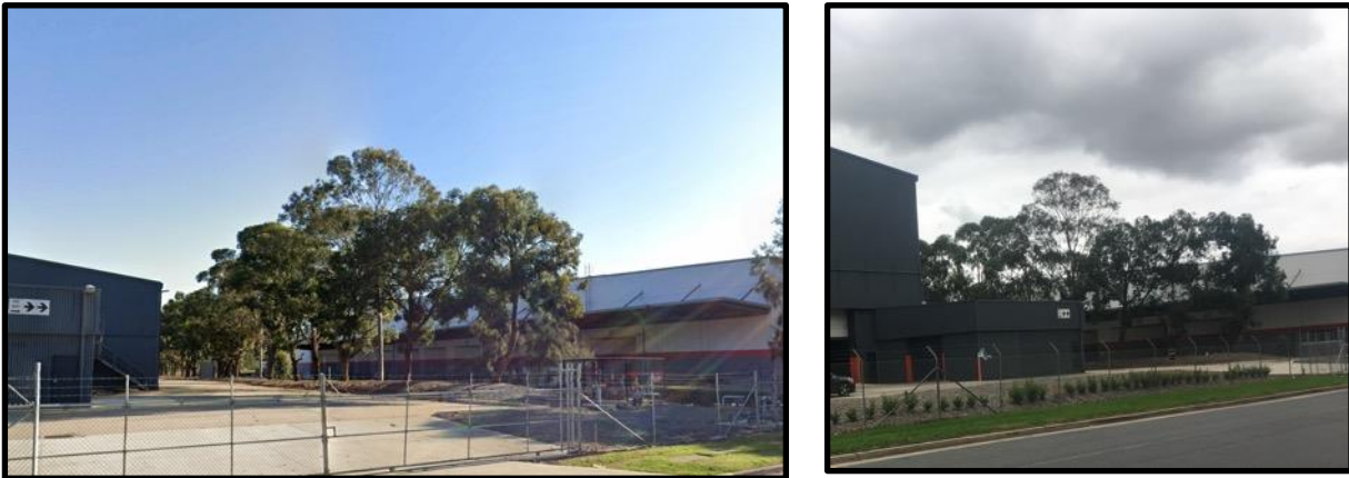
Figure 5: Looking towards the subject site for the proposed works which are the subject of the current 4.55 Application - as viewed from Loftus Road (Source: Concise Planning Pty Ltd, 2020, Google, 2021)
