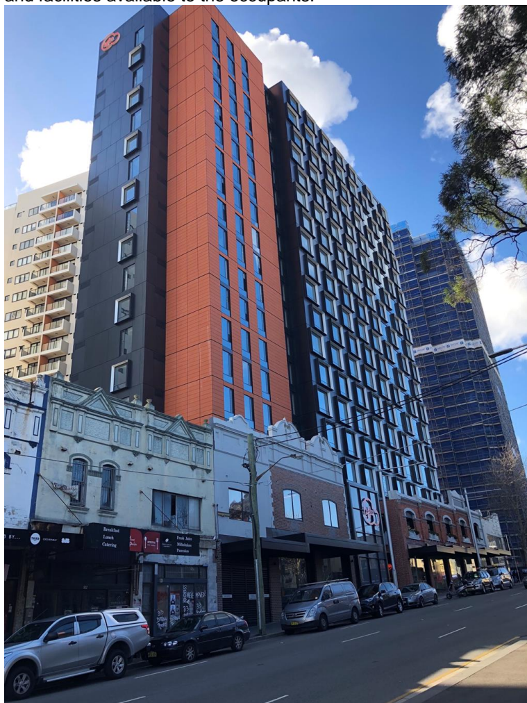
Figure 1 Iglu Redfern at 68-70 Regent Street looking north east as viewed from Regent Street
