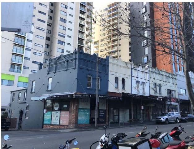
Figure 5 Existing buildings looking north west from Regent Street
