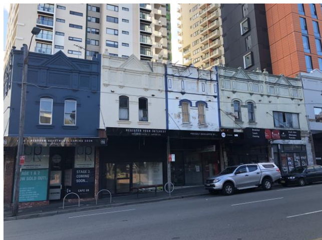
Figure 6 Existing buildings looking west from Regent Street
