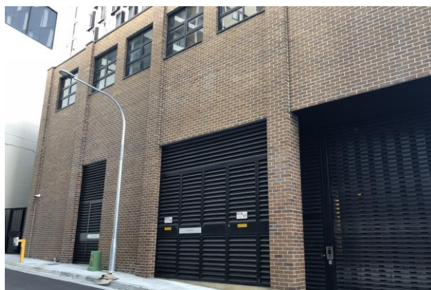
Figure 10 Secured access between William Lane and secured
