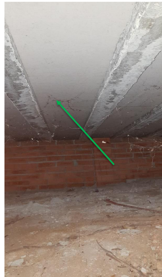
Photograph 9: B00L Subfloor – Compressed fibre cement sheeting – No Asbestos detected ( WSP-050264 )
