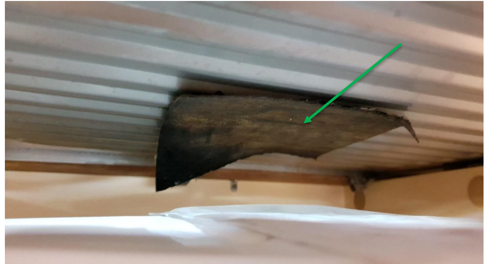
Photograph 7: B00E R0005 – Membrane beneath sink – No Asbestos detected (WSP-050262)
