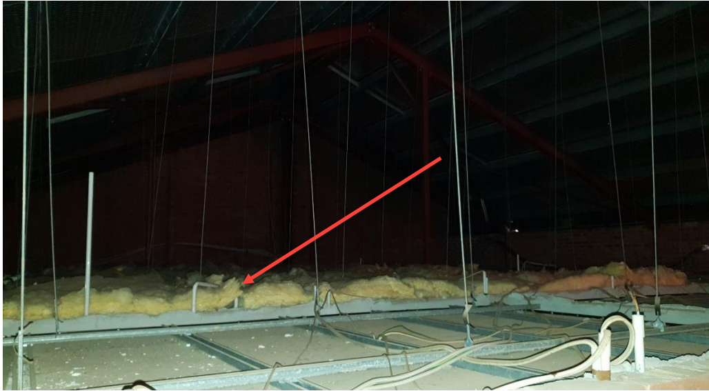
Photograph 4: B00B - Ceiling space – SMF ceiling batts
