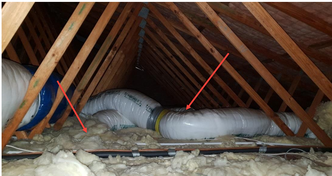
Photograph 8: B00L Ceiling Space– SMF ceiling batts as well as A/C ducting
