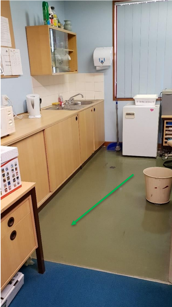
Photograph 6: B00E R0005 - Green vinyl floor lining – No Asbestos detected (WSP-050263)
