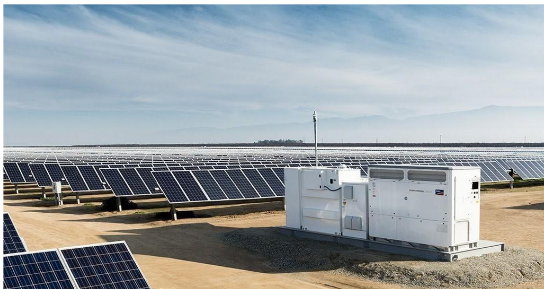
■ Figure 3. 9 Power conversion unit (Source: SMA)
