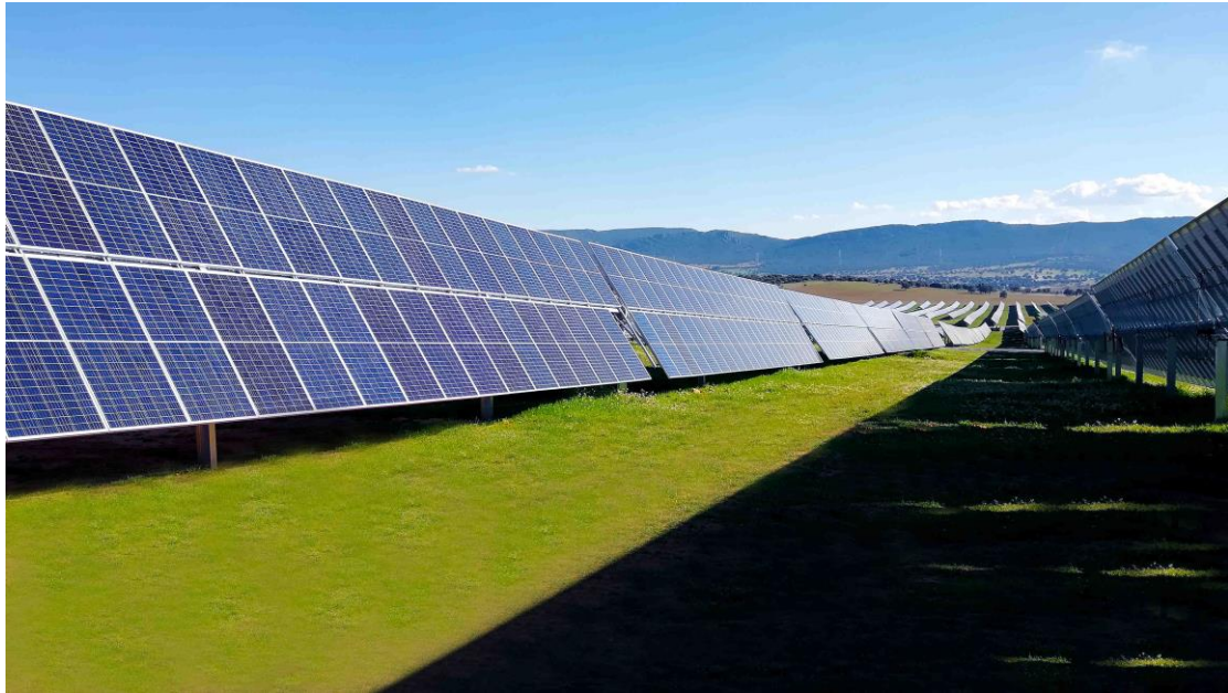
■ Figure 3.7 Single axis tracker with two panels in portrait (Source: Arctech Solar)
