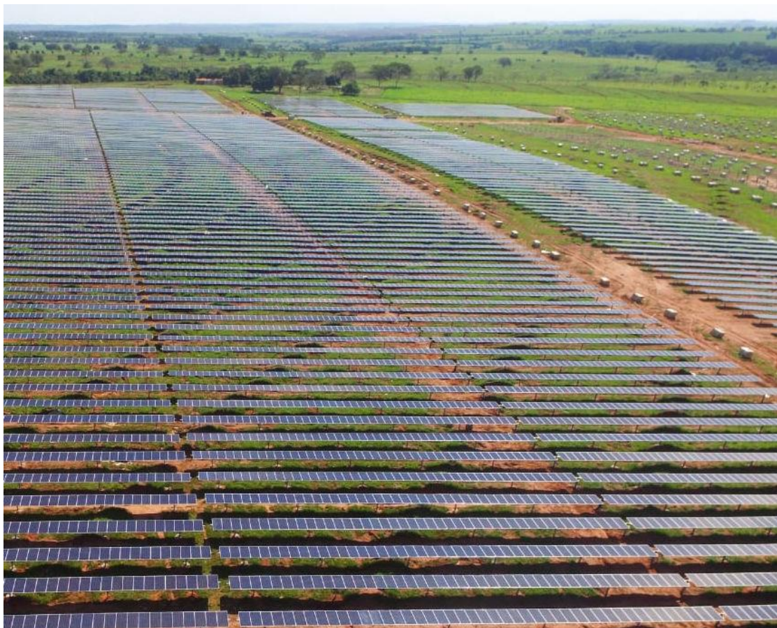
■ Figure 3.8 Single axis trackers with one panel in portrait (Source: Arctech Solar)
