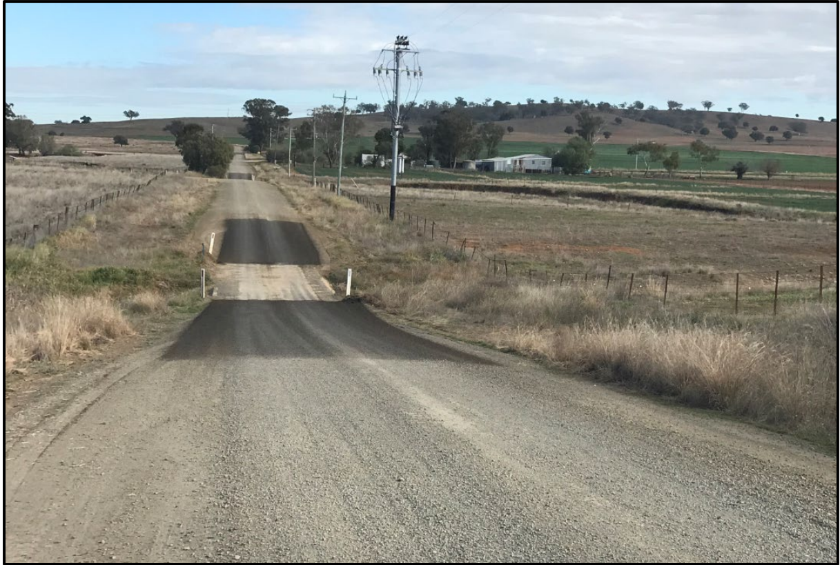
Photo 4 – Water crossing on Babbinboon Road showing sealing on approaches
