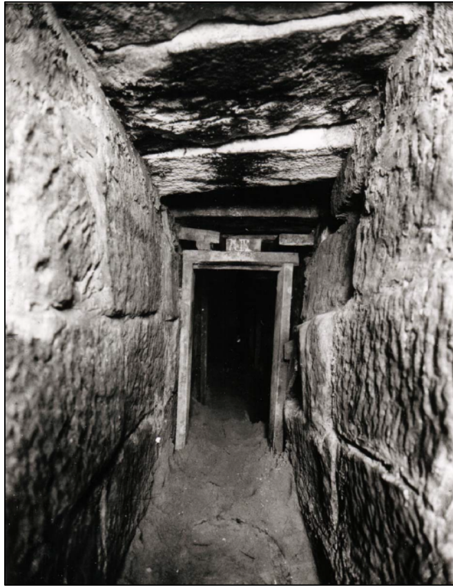
FIGURE 8: SECTION OF BUSBY'S BORE NEAR INTERSECTION OF LIVERPOOL AND COLLEGE STREETS, THIS SECTION OF THE BORE WAS CONSTRUCTED AS AN OPEN CUT TRENCH, LAID WITH SANDSTONE MASONRY AND SLAB ROOF (SOURCE: SYDNEY WATER ARCHIVES, REF: A1029)
