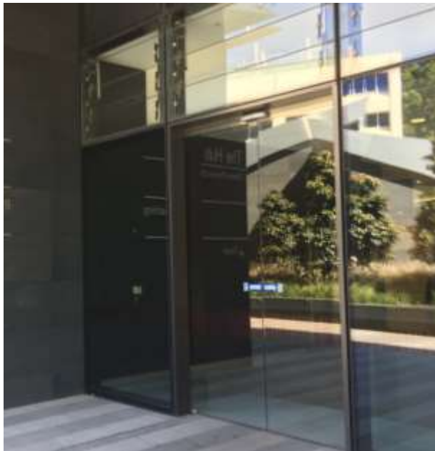
Luminance contrast is not achieved due to glare and shadow cast as well as the reflective nature of the selected glass.
