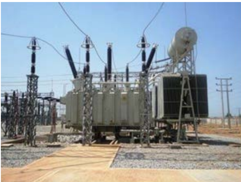
Photo 6 Typical 350MVA Transformer
