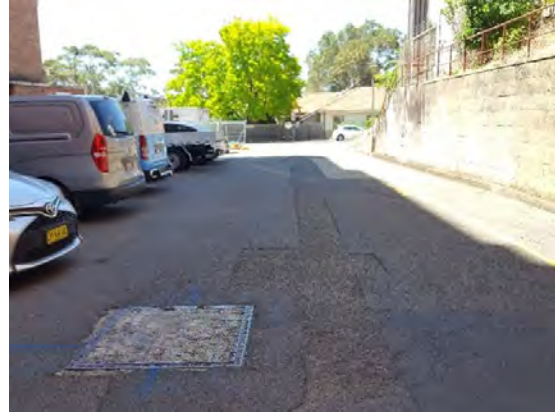
Photo 2. Looking south across loading dock with concrete cuts noted running parallel with loading dock access road.
