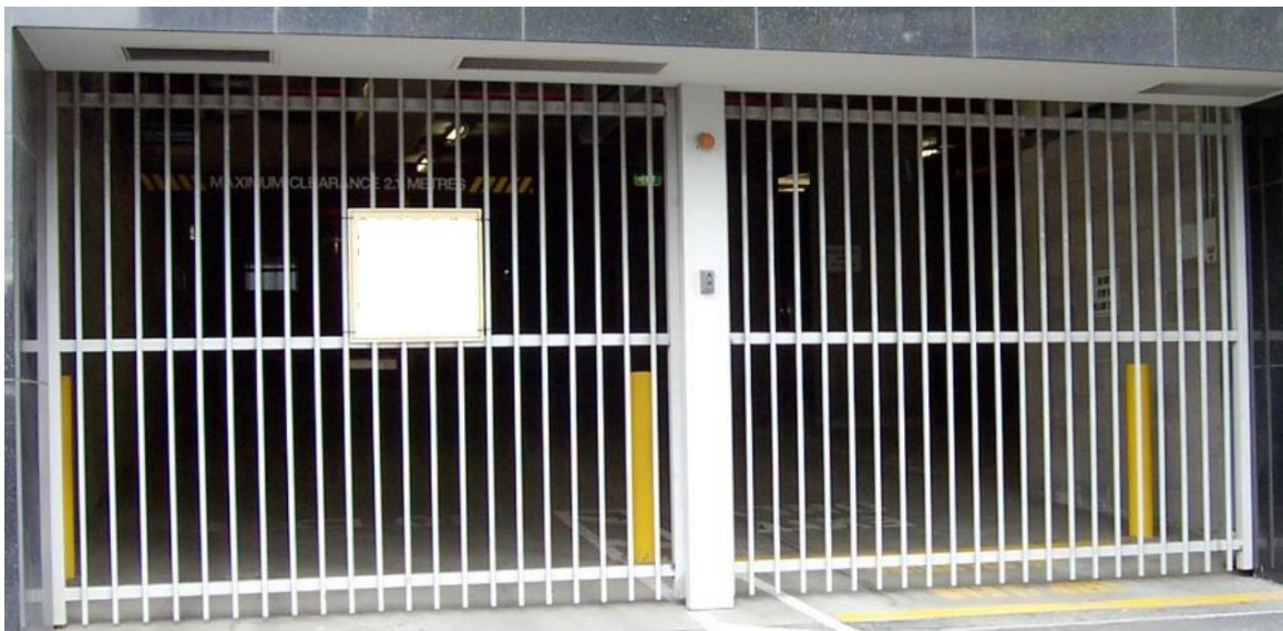
Figure 7 - Example of Basement Carpark Dual Sliding Security Gates
