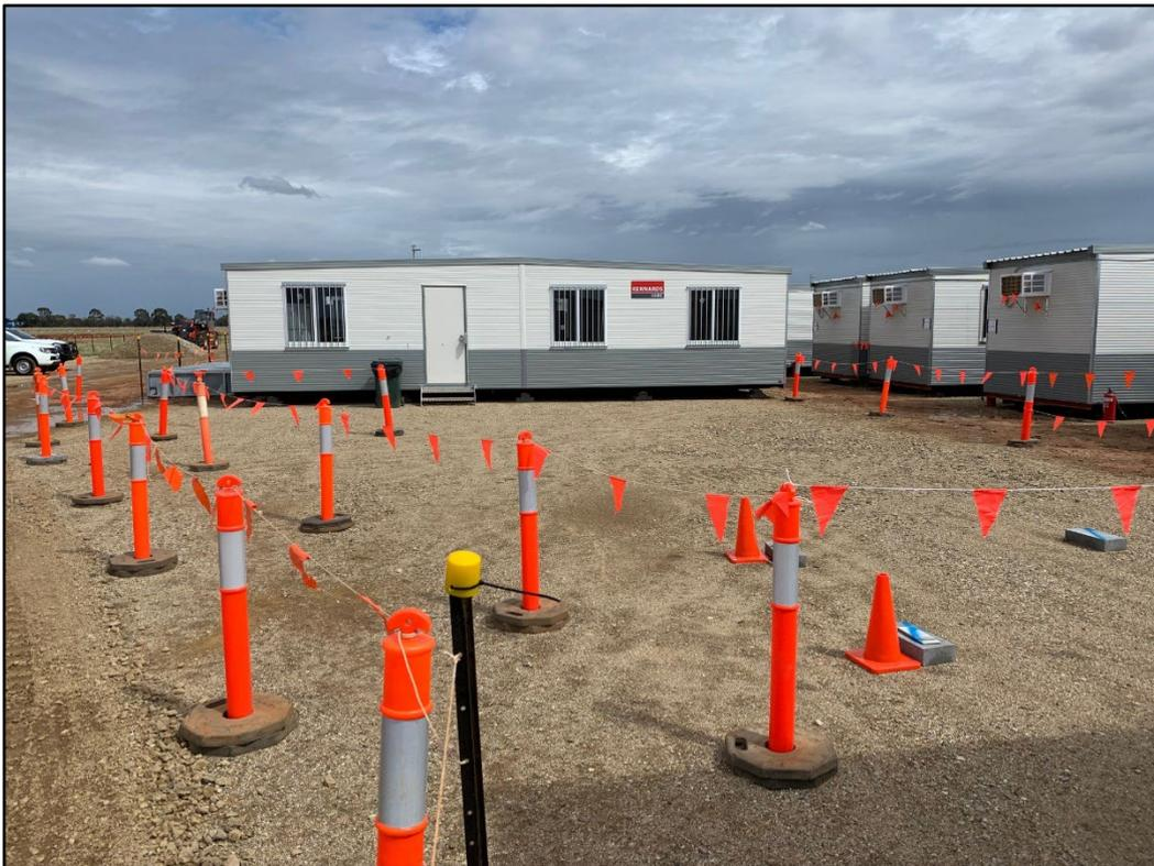
**Plate 5:** View of the main site compound and surrounds showing gravel hardstand area constructed to reduce potential for erosion and/or sedimentation in this area.
