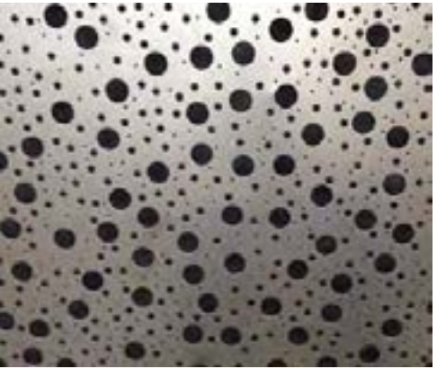
Perforated Steel to Step Risers for aeration & natural light (powder-coated dark grey - black colour)
