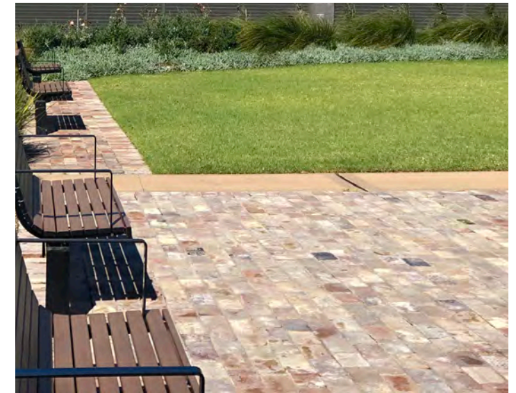
Recycled Brick Paving
