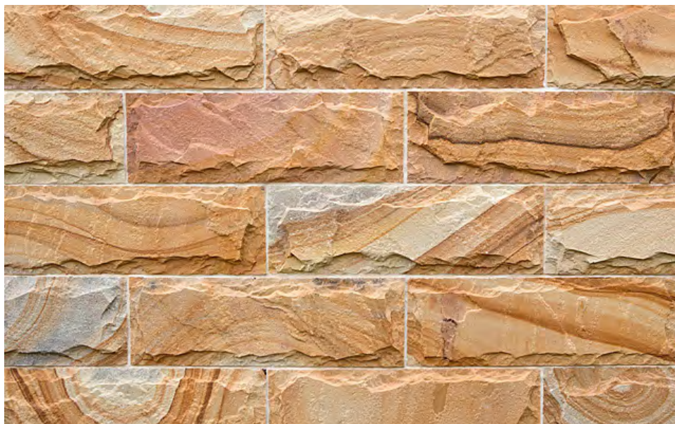
Sandstone Retaining Wall
