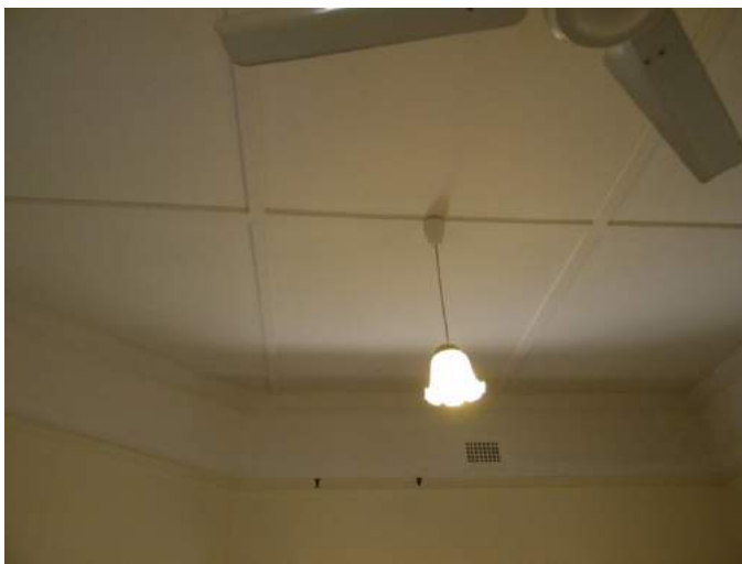
Figure 157: Typical battened ceiling and picture rail. Figure 158: Bay window.
