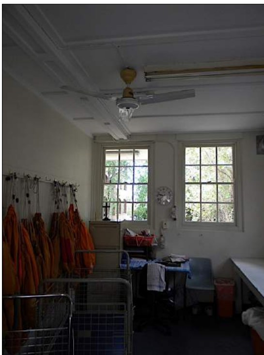
Figure 140: Typical ground floor room with battened ceiling and simple timber joinery. It would appear that the interior wall has been moved from its original location.
