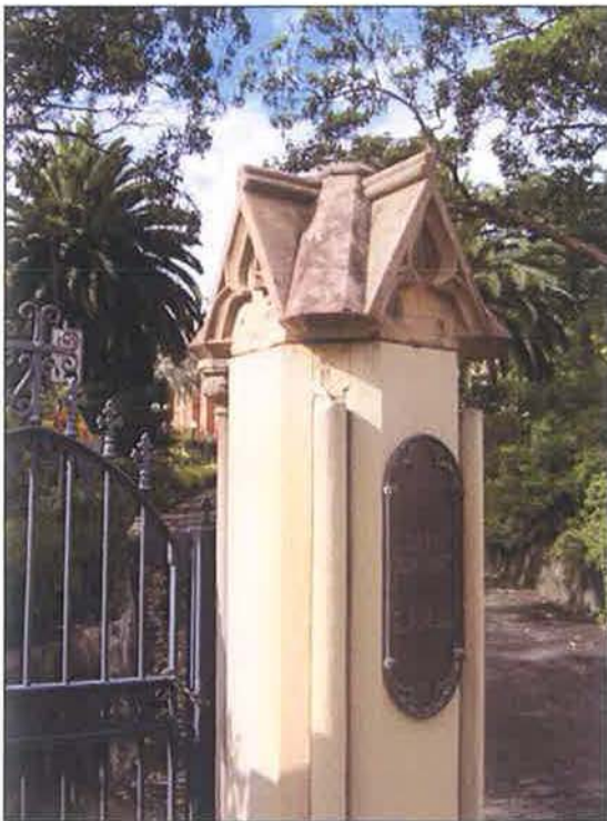
Figure 3.13 Detail of one of the posts. The capping appears to be original with a patina of age. The shaft and base may have been replaced and differ in colour. The piers appear to be sound, however, some of the decorative detail is missing and some of the stone on the capping has been chipped and is fretting.
