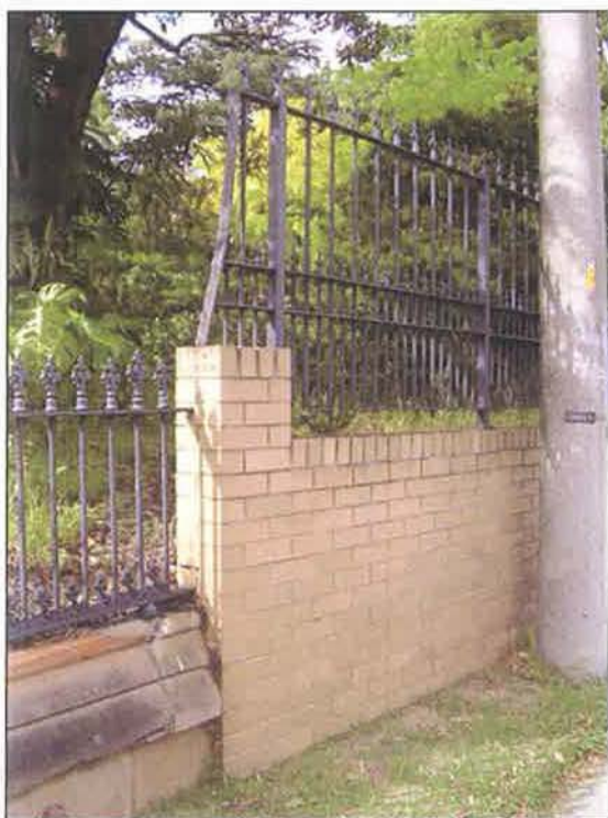
Figure 3.16 The junction of the original sandstone fence and more recently constructed fence extending along the western section of the Pennant Hills Road boundary. The blond brick base of the fence forms a retaining wall along this section of the site.
