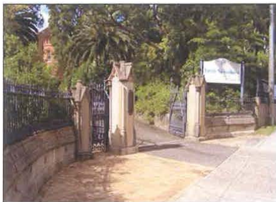
Figure 3.8 The original sandstone gateway located on the Pennant Hills Road frontage. The gates are setback from street kerb and retain what it assumed to be the original wrought iron palisade fencing and gates.
