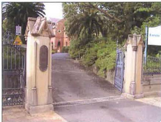
Figure 3.9 An asphalted driveway extends from the gates to the original main building. The driveway is flanked by two sandstone piers with gothic styled carved details and capping. The piers support the driveway wrought iron gates and separate pedestrian gate (at left). The posts and gates are framed by a wrought iron palisade fence on a sandstone base which also features decorative mouldings and religious motifs.
