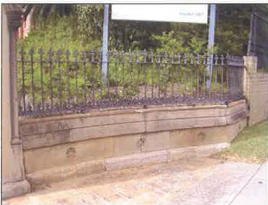
Figure 3.14 The western section of the original gateway and fence. The stone appears to be sound, however, some damage, chipping, fretting and discolouration is evident along its length.
