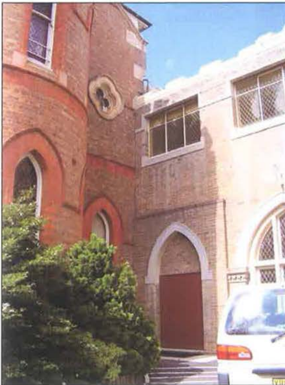
Figure 3.74 Detail of the junction between the 1897 building and 1953 Chapel. The building also features castellated parapet, pointed arched openings with profiled mouldings on the ground floor and leaded windows.
