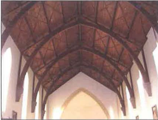
Figure 3.80 Detail of the timber Chapel ceiling.
