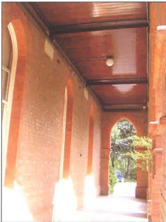
Figure 3.59 The ground floor verandah features simple concrete slab and timber boarded, bayed ceiling which appears to be in good condition and well maintained.
