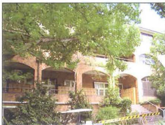
Figure 3.86 Part of the eastern façade of the Mary Ward Wing. The building is a three storey building over basement constructed of face bricks with hipped terracotta roof clad in tiles. Open verandahs extend along the east and western facades of the building.
