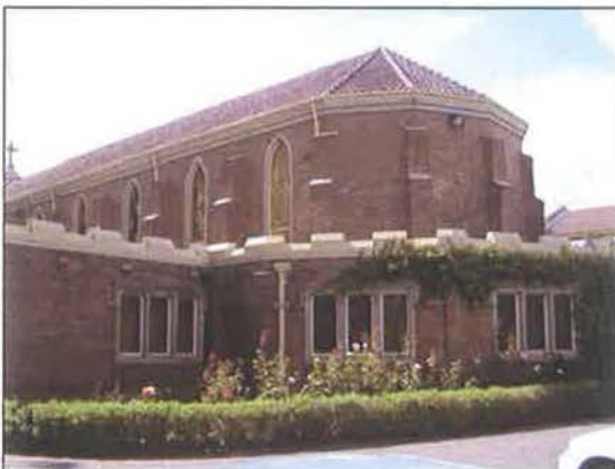
Figure 3.77 The Chapel features a gabled roof clad in terracotta tiles with faceted hip over the curved western end. Buttresses/engaged piers also delineate the bays of the building. Each bay also features a set of leadlight windows with stone surround.
