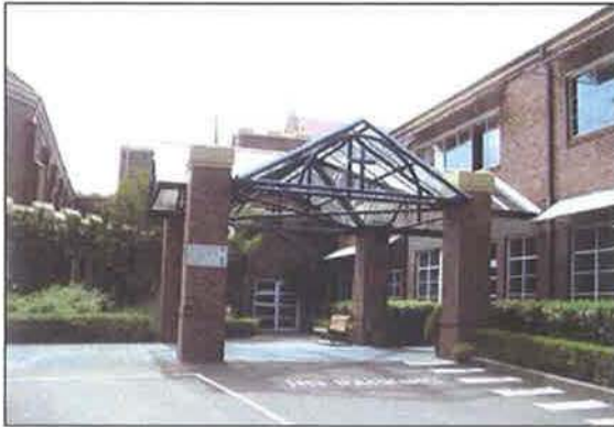
Figure 3.111 Entry to the main office is marked by a modern steel framed roof supported on brick piers dating from 1992. Note the Holy Angels Wing at rear.
