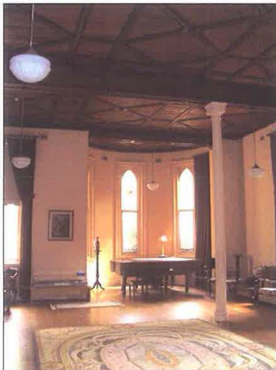
Figure 3.60 The interior of original classroom, now used as a reception room. The room features timber floors, rendered and set walls, timber joinery including deep profiled skirtings and profiled architraves and lead light windows. Note the cast iron columns and decorative timber ceiling.
