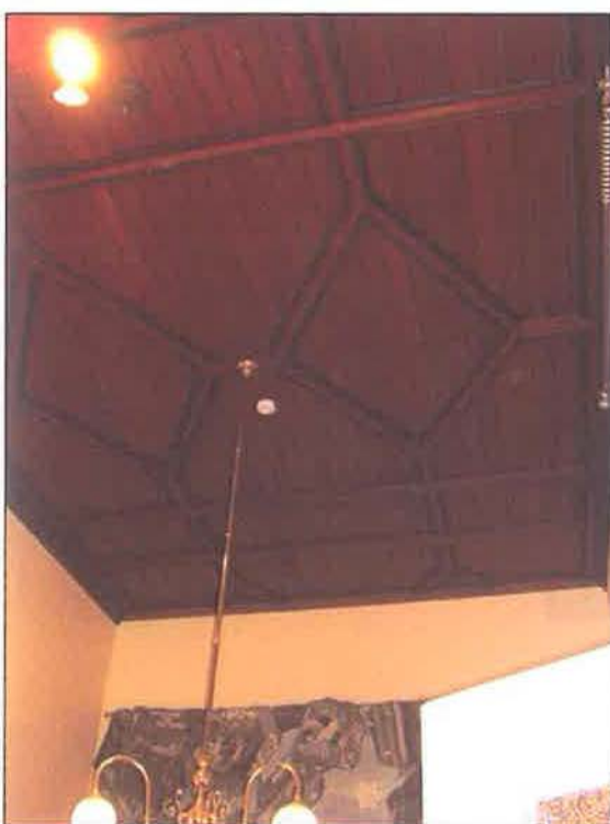
Figure 3.66 Detail of the timber boarded ceiling in the Brewer Room.
