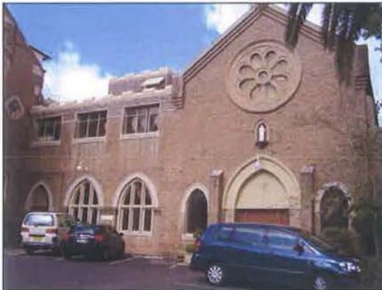
Figure 3.73 The 1953 Chapel building and cloister is constructed of face brick with rendered and stone details. The main entry is surmounted by a prominent gable with decorative stepped and rendered gable cap over the rose window.
