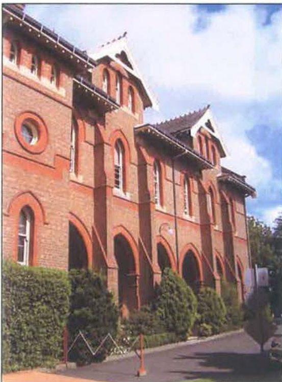
Figure 3.57 The eastern façade of the 1897 building which features open verandah on the ground floor and other features typical of the style and works of Hennessy including wall buttresses that delineate the building bays, pointed arched openings and distinctive dormer windows.
