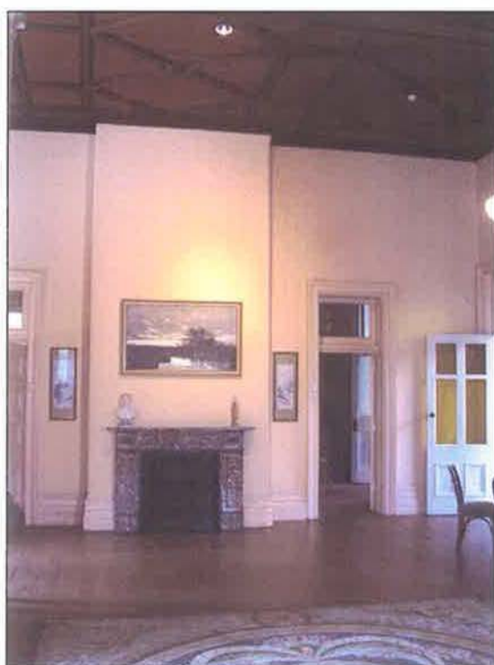
Figure 3.61 The southern wall also features a chimney breast with marble fireplace surround and cast iron grate and ceramic tiled hearth.
