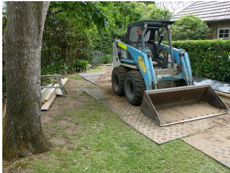
Figure 4 – Showing typical detail for truck mats.
