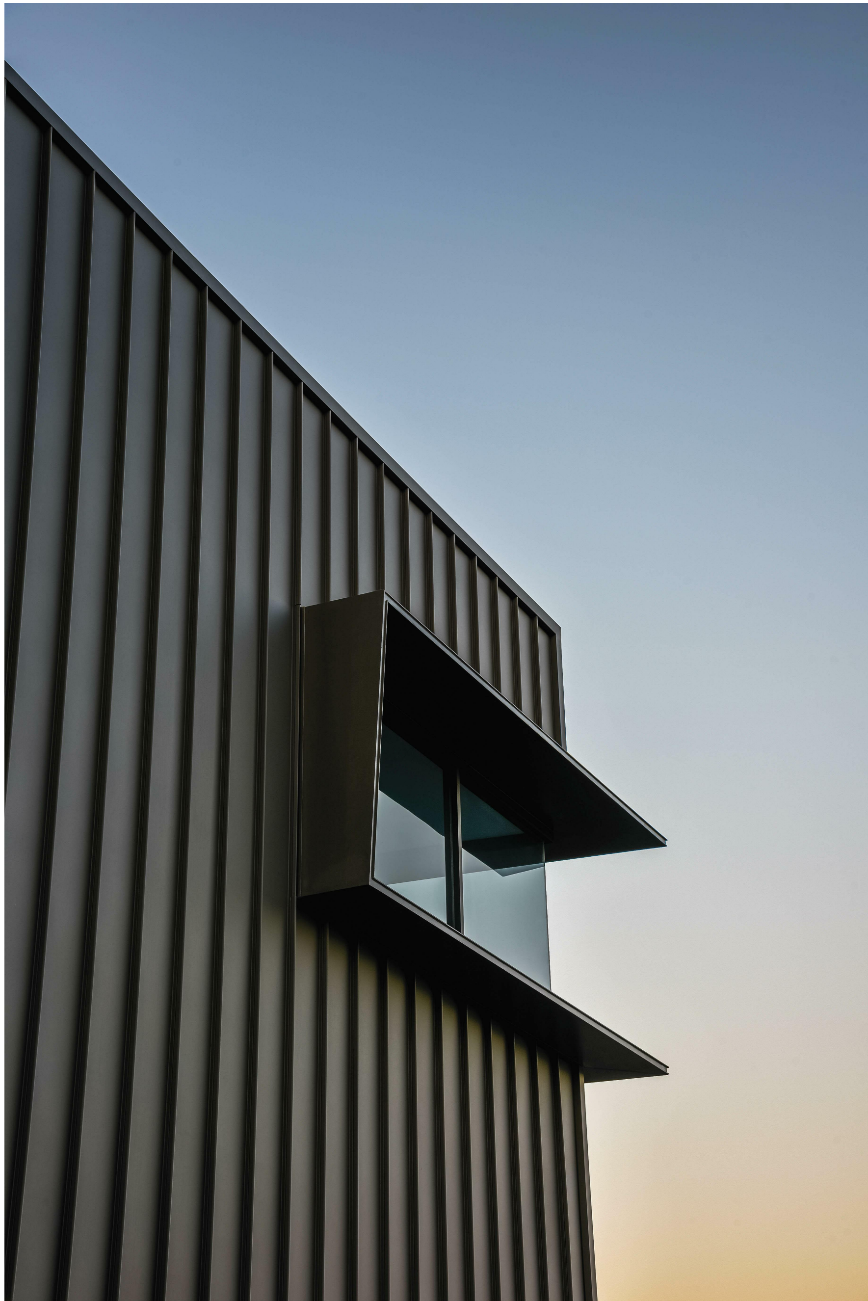
EWC 2 - EXTERNAL WALL CLADDING 2
