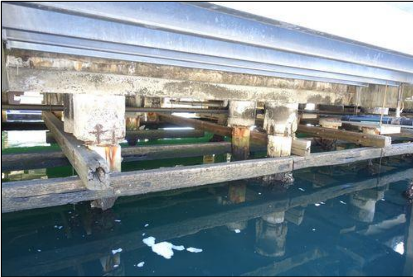
Photograph 7: Blackwattle Bay Marina B2 showing timber pylons and bracing beams
