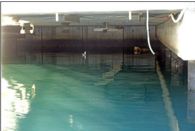
Photograph 6: Underside of the reinforced concrete deck of the wharf east of the coal loader showing seawall that runs the length of the site about 20m from Bridge Road.
