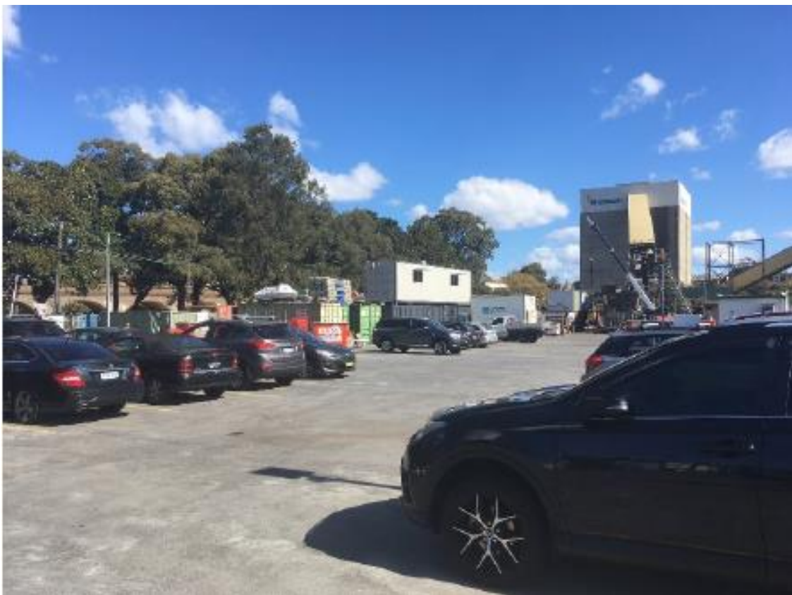
Figure 5 | View of the site looking south west (source: EIS)
