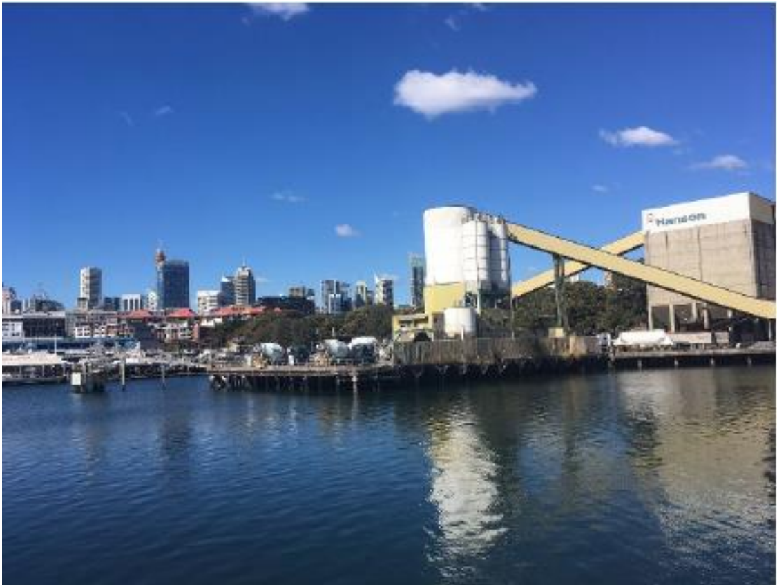
Figure 6 | View of the site looking south east (source: EIS)
