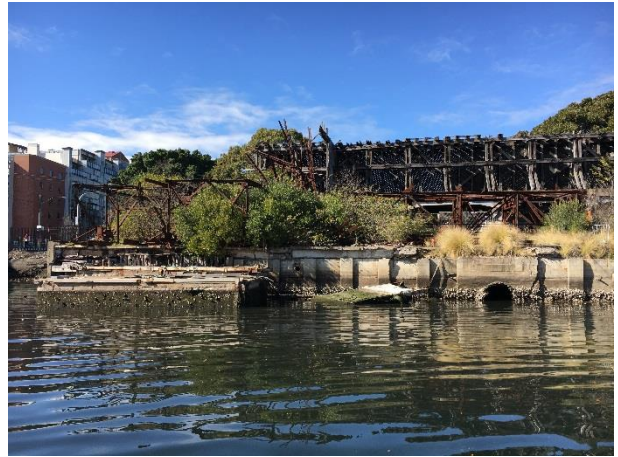
Stormwater outlet with oyster growth
