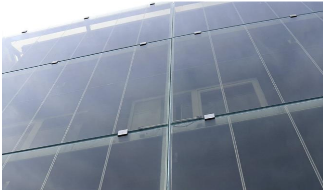
Figure 6: Onyx integrated solar façade. Source: Onyx Solar
