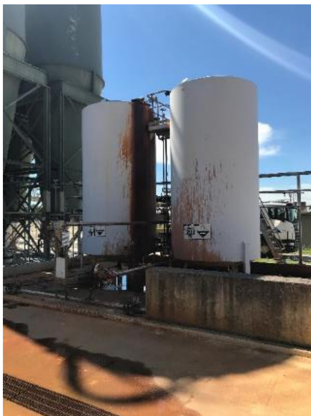
Photo 2-14: Existing ferric chloride tanks within the Lime Softening Plant
