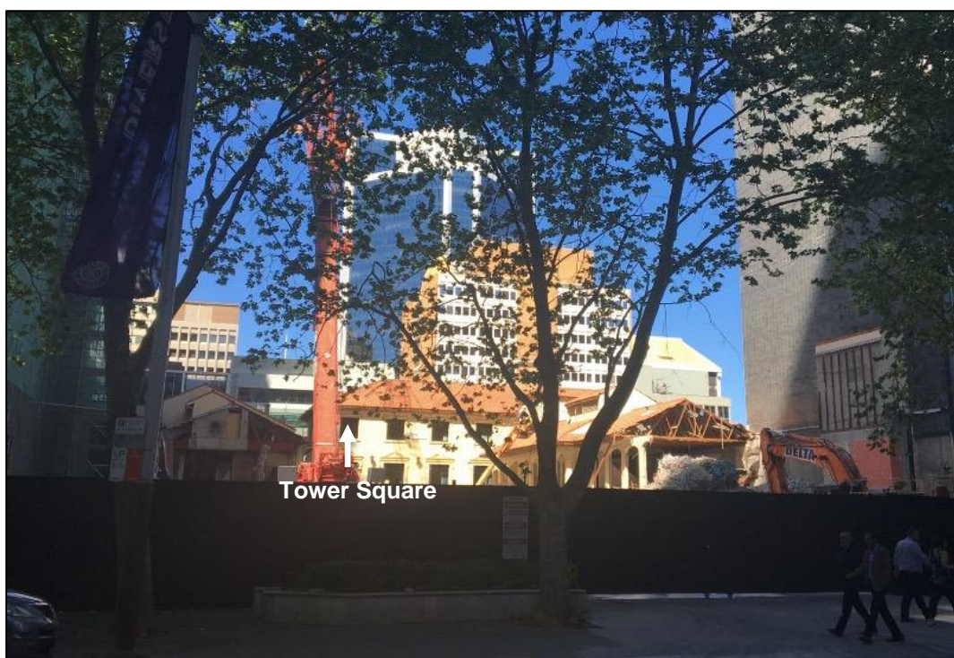
Figure 6 - Tower Square under demolition (seen from Miller St)
