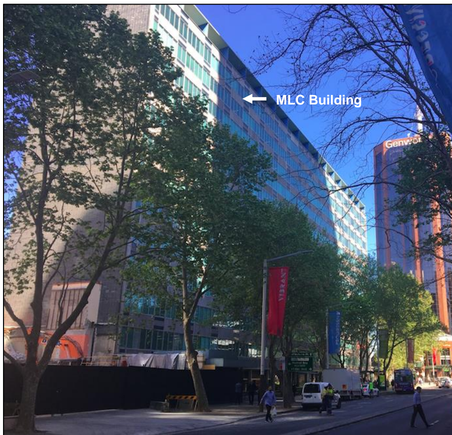
Figure 8 - MLC Building fronting Miller Street
