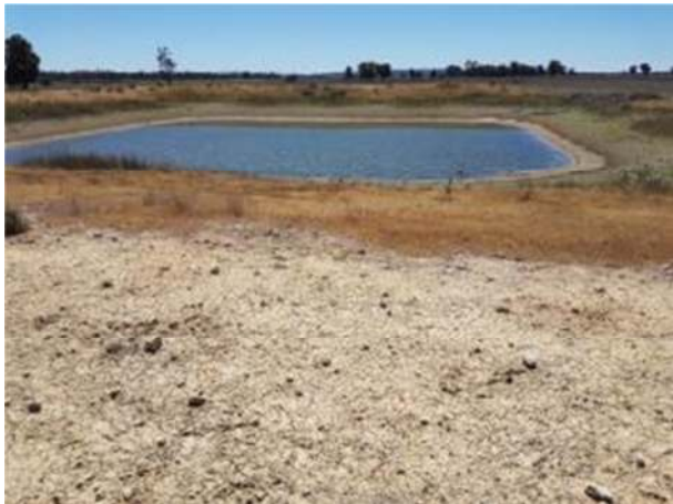
Plate 15. Dam on the Sandigo North property, showing the clay lining contrasting to the surrounding natural soils
