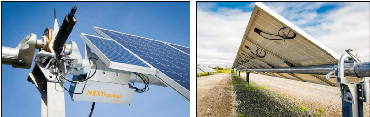
Figure 4-5 Example single axis tracking system (NexTracker)
