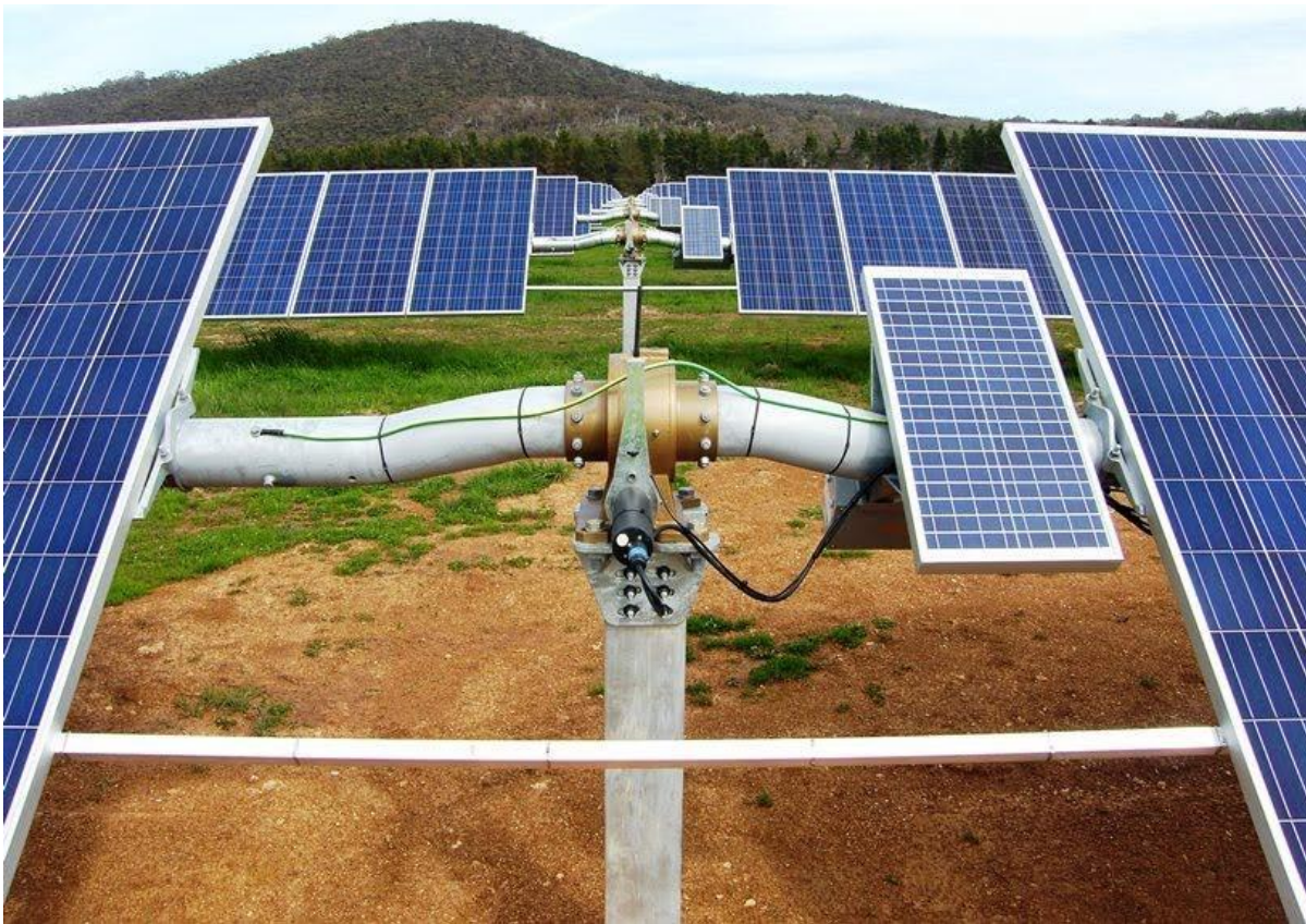
Figure 4-6 Example single axis mounting system from Mount Majura solar farm, ACT
