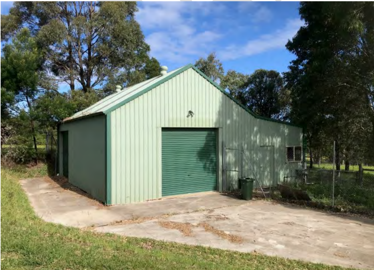
Photograph 10: a shed located in the south eastern portion of the site
