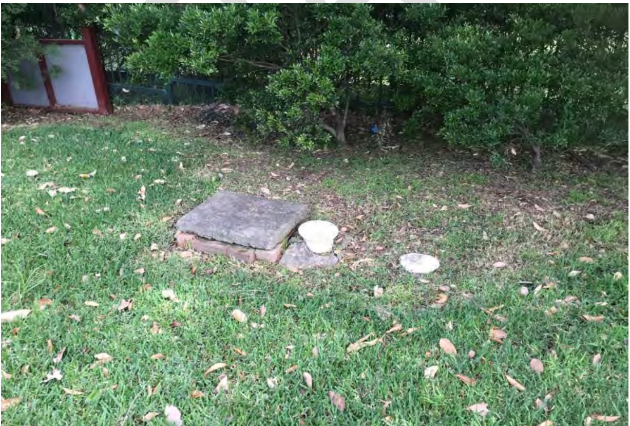
Photograph 20: a wastewater inspection point located in the vicinity of the existing preschool
