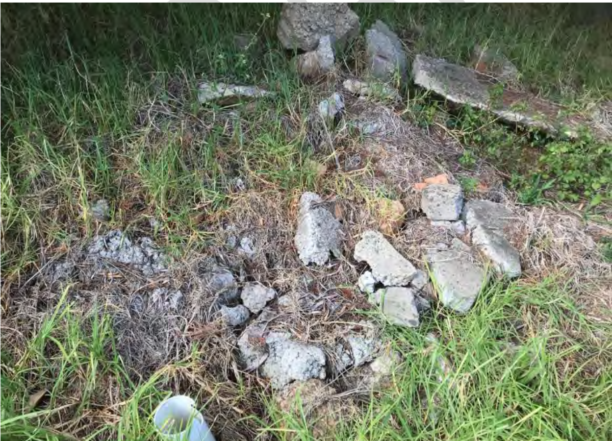
Photograph 8: a pile of demolition rubble observed in the south eastern portion of the site along the eastern boundary
