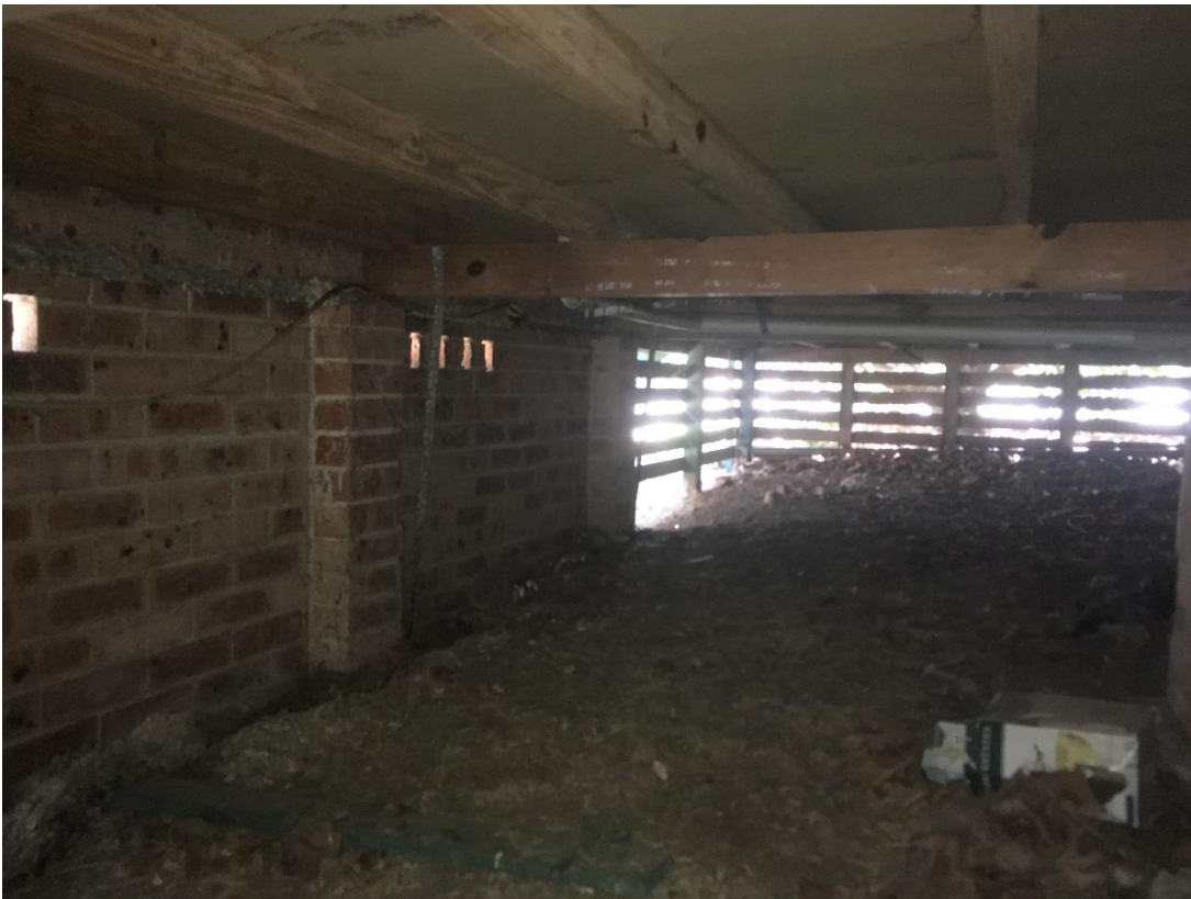
Plate 12: Space beneath one of the buildings to be demolished
