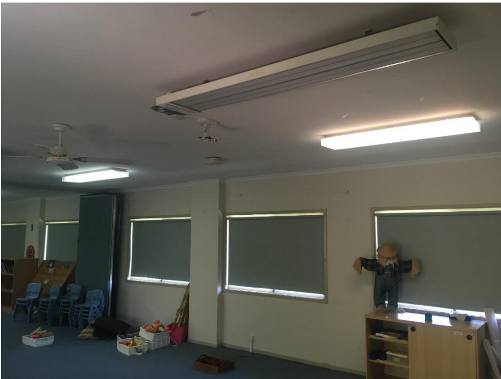
Plate 10: Gaps between light fitting were inspected for evidence of use
