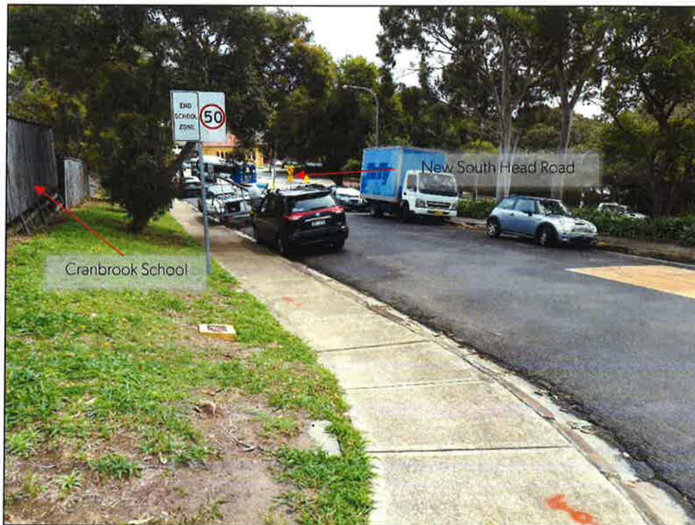
Figure 12 | View towards Rose Bay Avenue and New South Head Road intersection (Source: DP&E 2018).
