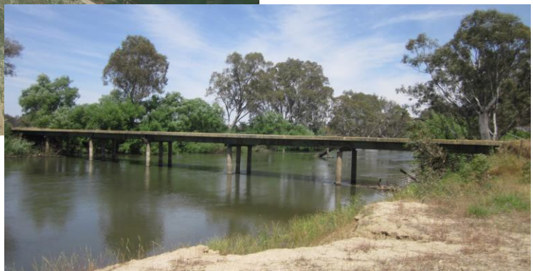
Photo #1 Looking west from north side
