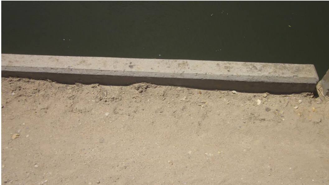
Photo #10: Edge kerbing and drainage slots
