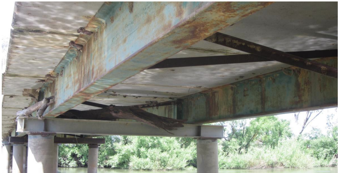
Photo #3 Underside of bridge deck showing main 610UB beams and lateral braces; cross head beams 250UC and piles
