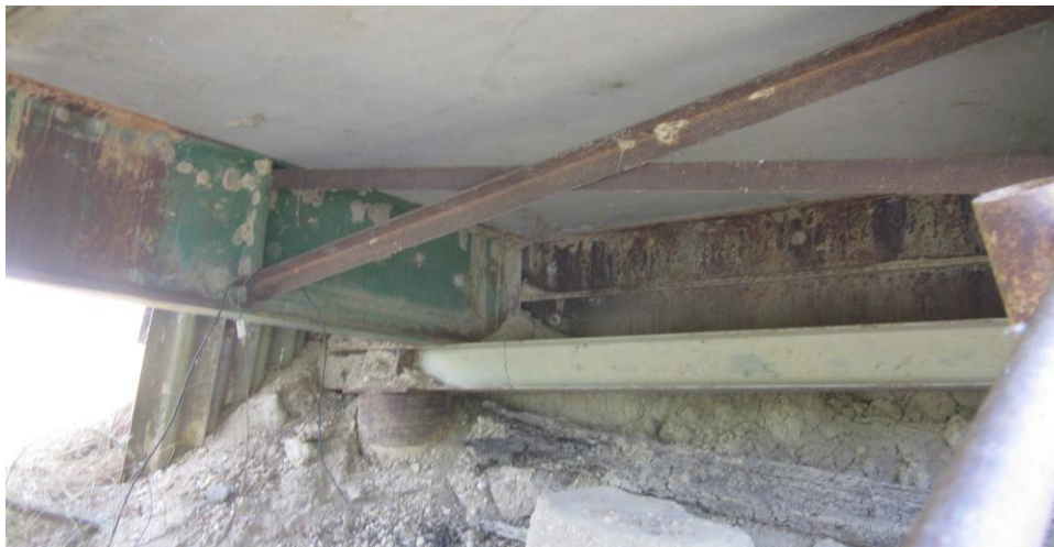
Photo #7: Edge foundation- North abutment
