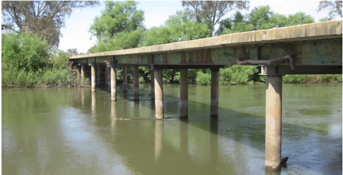
Photo #2 Looking west from north embankment
