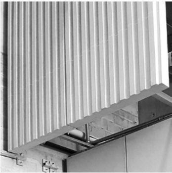
CON-02 Glass Reinforced Concrete Panels (GRC) Colour: Colour: Acid Wash with Micro Aggregate Finish
