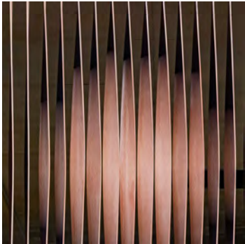
SCN-01 Aluminium Vertical Battens (Modulated Spacing) Finish: Red/Brown (to match PLC Carpark)
