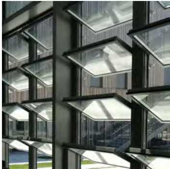
CODE REFERENCE: LVR-01 DESCRIPTION: Operable Acoustic Glazed Louvres with Aluminium Framing MATERIALS AND COLOURS: Finish: Clear/Black
