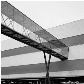
GL-02 / STL - 02 Structural Glazing with Steel Subframing Finish: Clear/Black Framing
