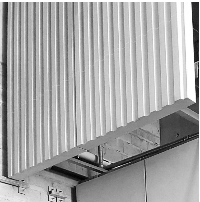
CODE REFERENCE: CON-02 DESCRIPTION: Glass Reinforced Concrete Panels (GRC)
