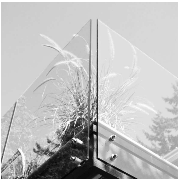
CODE REFERENCE: BAL-02 DESCRIPTION: Glazed Frameless Balustrade
