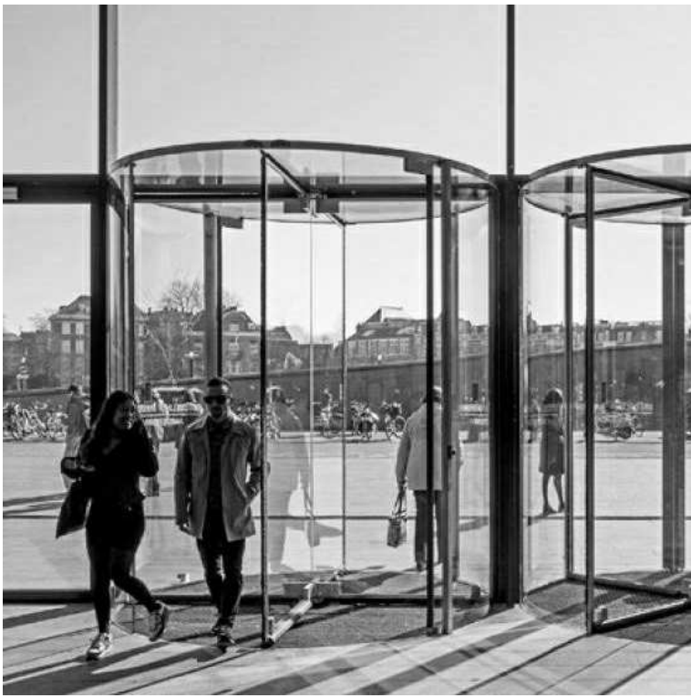
CODE REFERENCE: DT-01 DESCRIPTION: Glazed Revolving Door
