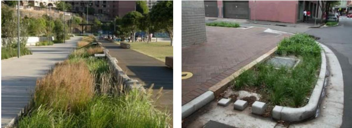
Figure 11: Bioretention system (raingardens) at Pirrama Park, Pyrmont (left), Chippendale (right) (Photos: Alluvium).
