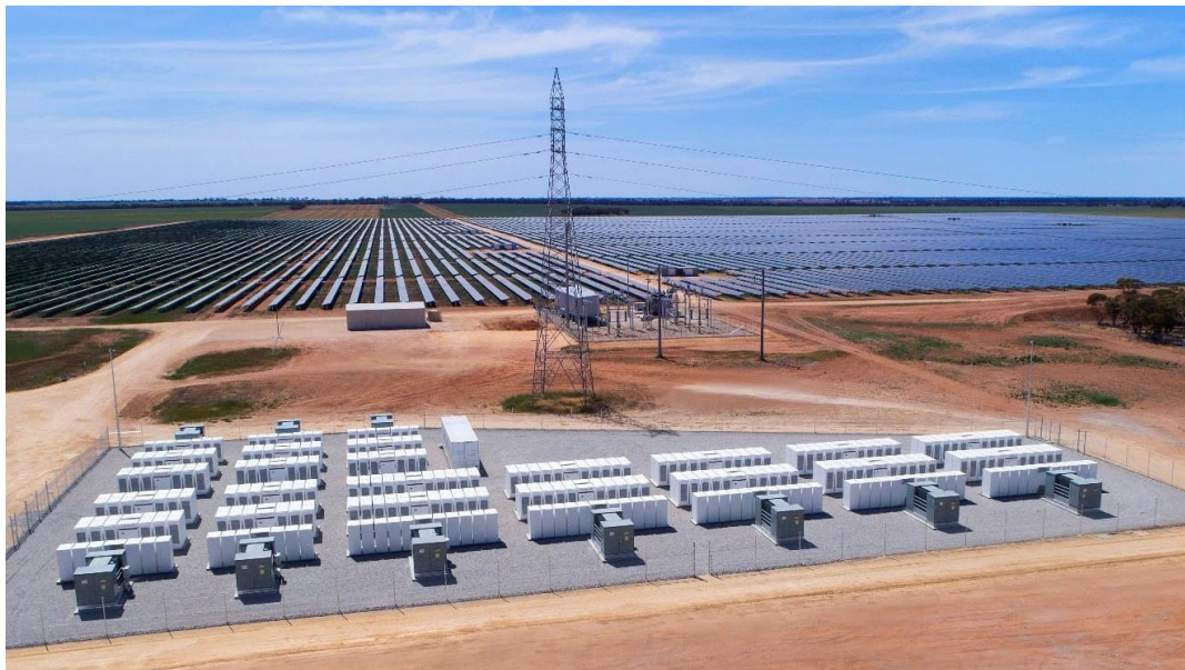
Image 1: Illustration of a Centralised BESS (referred to as format 1 in this report) coupled with a solar farm (5 times smaller than the Maryvale BESS) – for illustrative purposes only
