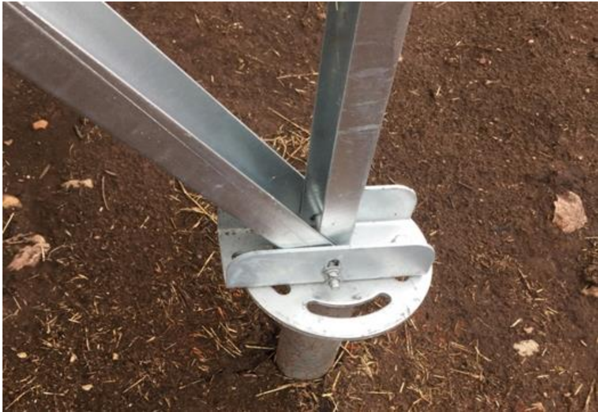
FIGURE 1 INDICATIVE SOLAR PANEL FOOTINGS
